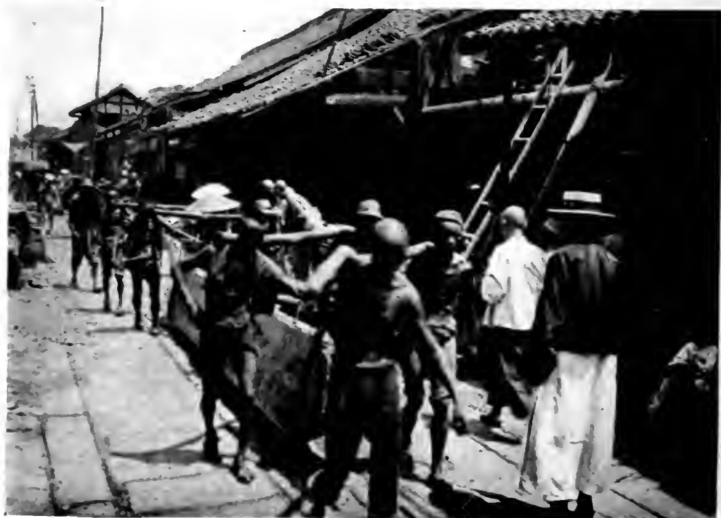
Perhaps some such method was used for carrying great stones during the building of the pyramids as this means of getting mammoth granite slabs where they were needed in Chengtu under renovation
